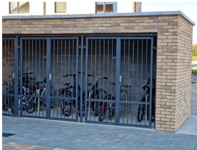
On street, secure bicycle store with Sheffield Stands; Reference Project: Woodbrook Phase 1, in DLRCC
